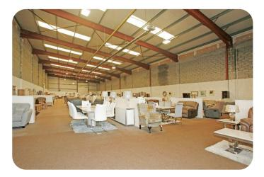
The building is of concrete frame construction with a steel frame metal deck double skin insulated roof incorporating perspex roof light panels. The exterior walls are of concrete block wall construction inner and outer leaf at lower level, the unit incorporates vertical profile cladding from ground to eaves level externally.
